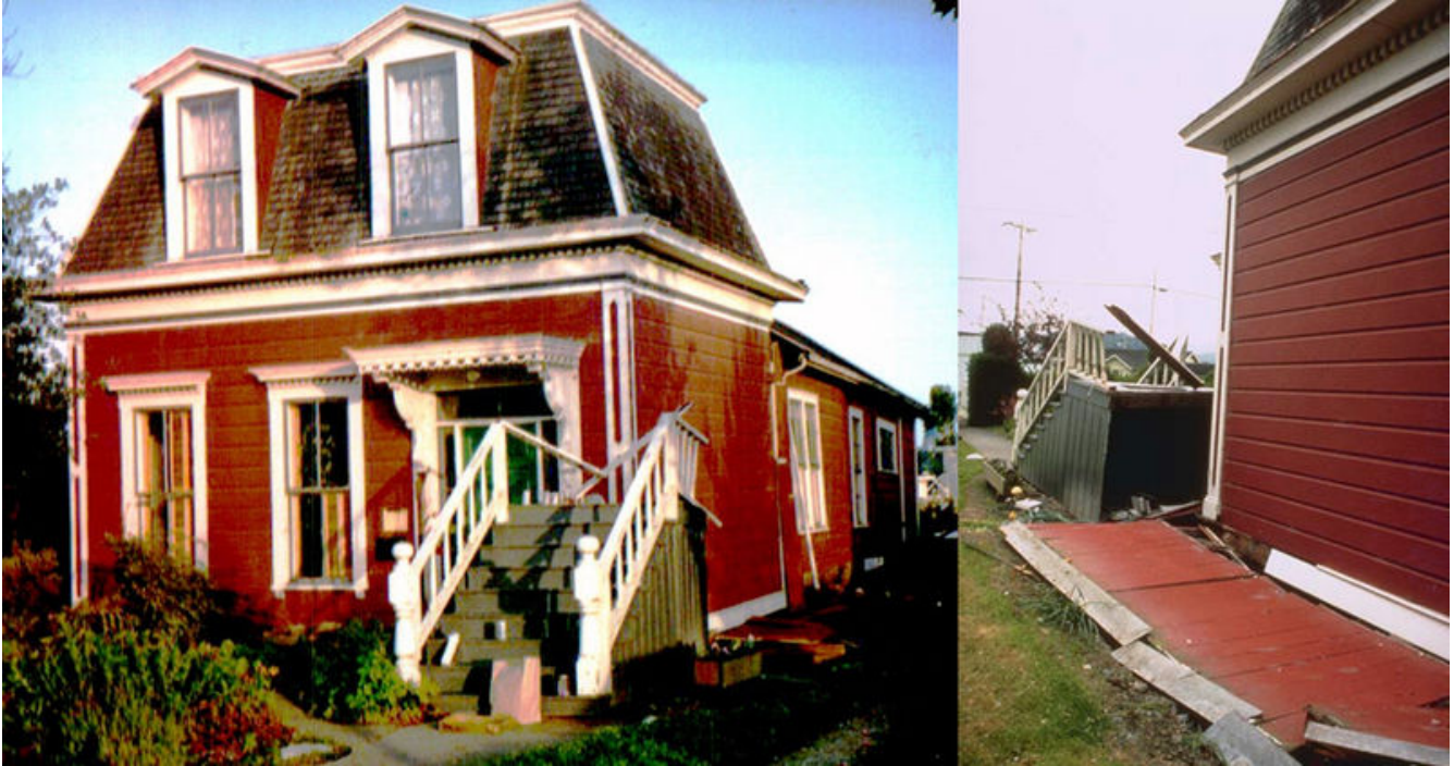
Figure 11-4. This Victorian wood-frame house in Ferndale, California, was built on a post-and-pier foundation, but was not bolted to its foundation, so that it slid off during the 1992 Cape Mendocino Earthquake. The floor level of the house was at the same height as the front steps. The house moved to the right and down with respect to the steps. The wooden skirting, formerly part of the outside wall, is now flat on the ground. Left-hand photo is view of house from front, and right-hand photo is view from one side. Photos courtesy of National Oceanic and Atmospheric Administration
