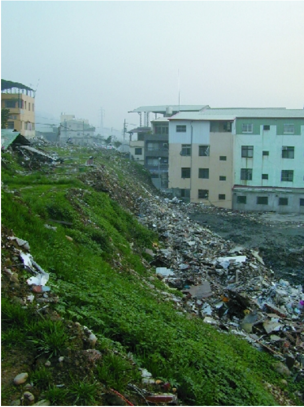
Figure 12-15. The Chi-Chi, Taiwan, earthquake was accompanied by surface rupture on the Chelungpu reverse fault. The photo is taken along the fault with the upthrown hanging wall on the left. The fault trace is between the two buildings in Fengyuan City, on which destruction was total. Photo by Charles Rubin, then of Central Washington University in Ellensburg.
