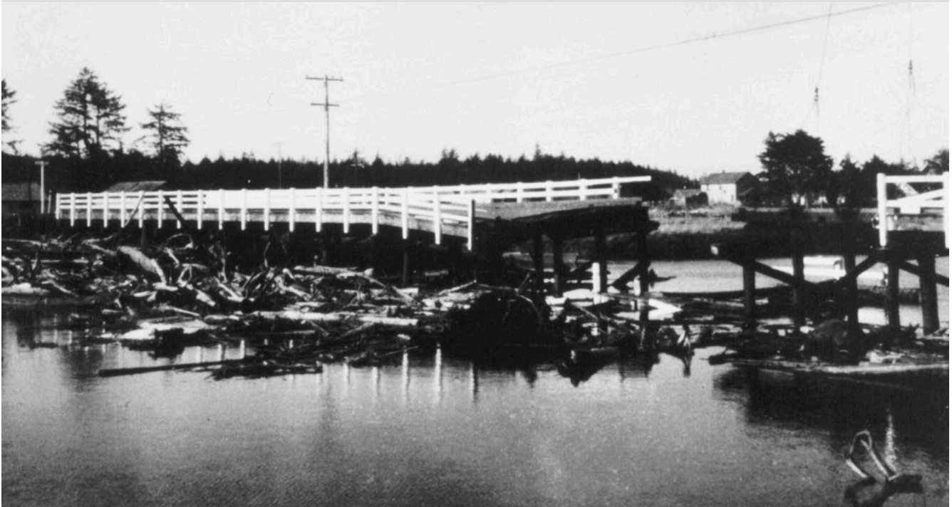
Figure 9-2. Bridge across Copalis River, Washington, destroyed during the tsunami accompanying the 1964 Good Friday Earthquake in southern Alaska.
