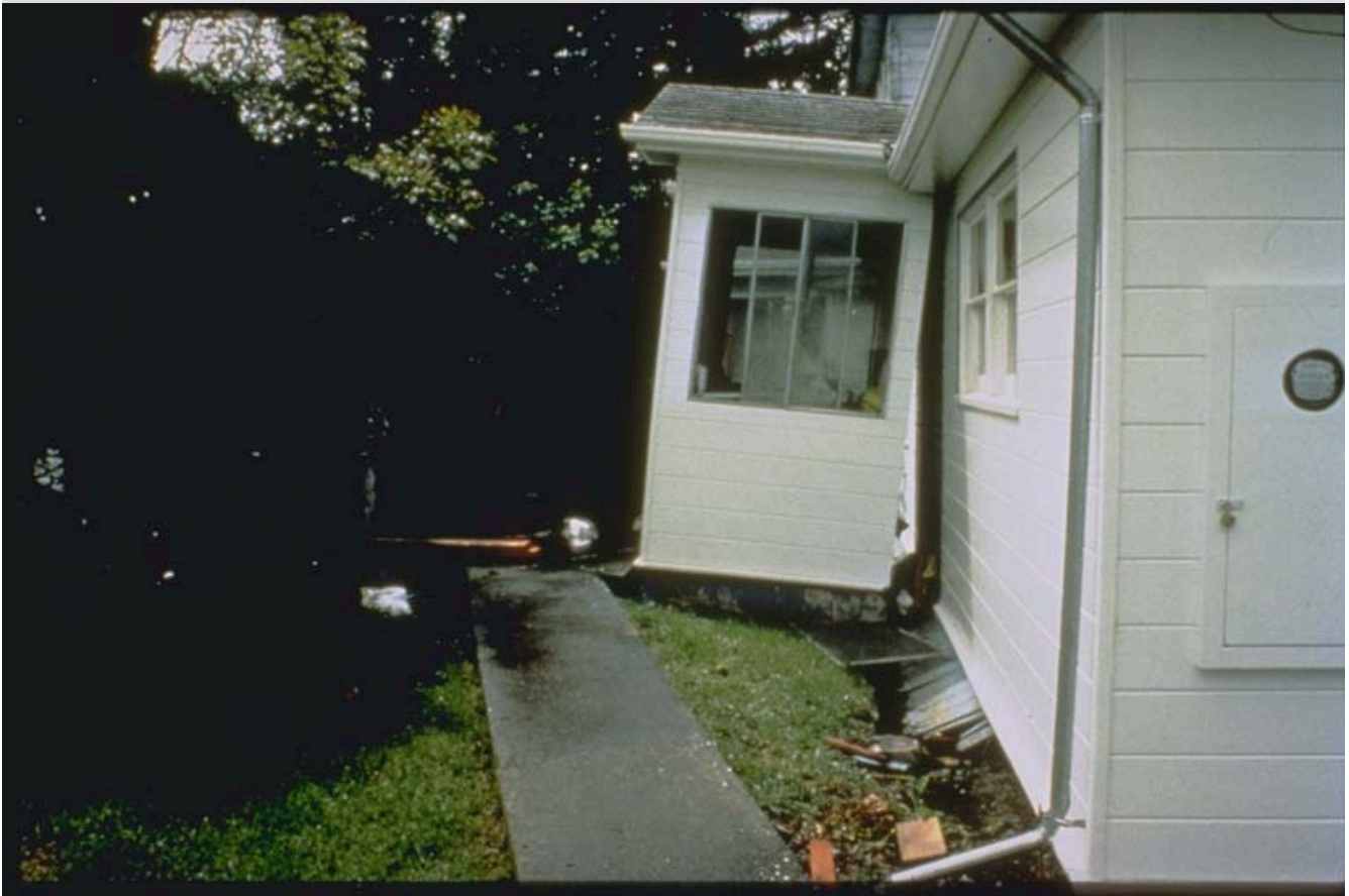
Figure 11-5. This house south of Petrolia, California, shifted off its foundation during the 1992 Petrolia Earthquake because it was not anchored to the foundation, and its cripple wall was not reinforced. The house shifted to the right, as seen by the collapsed wooden skirting. The separation of the house and the small porch is an example of connection failure. Photo courtesy of National Oceanic and Atmospheric Administration
