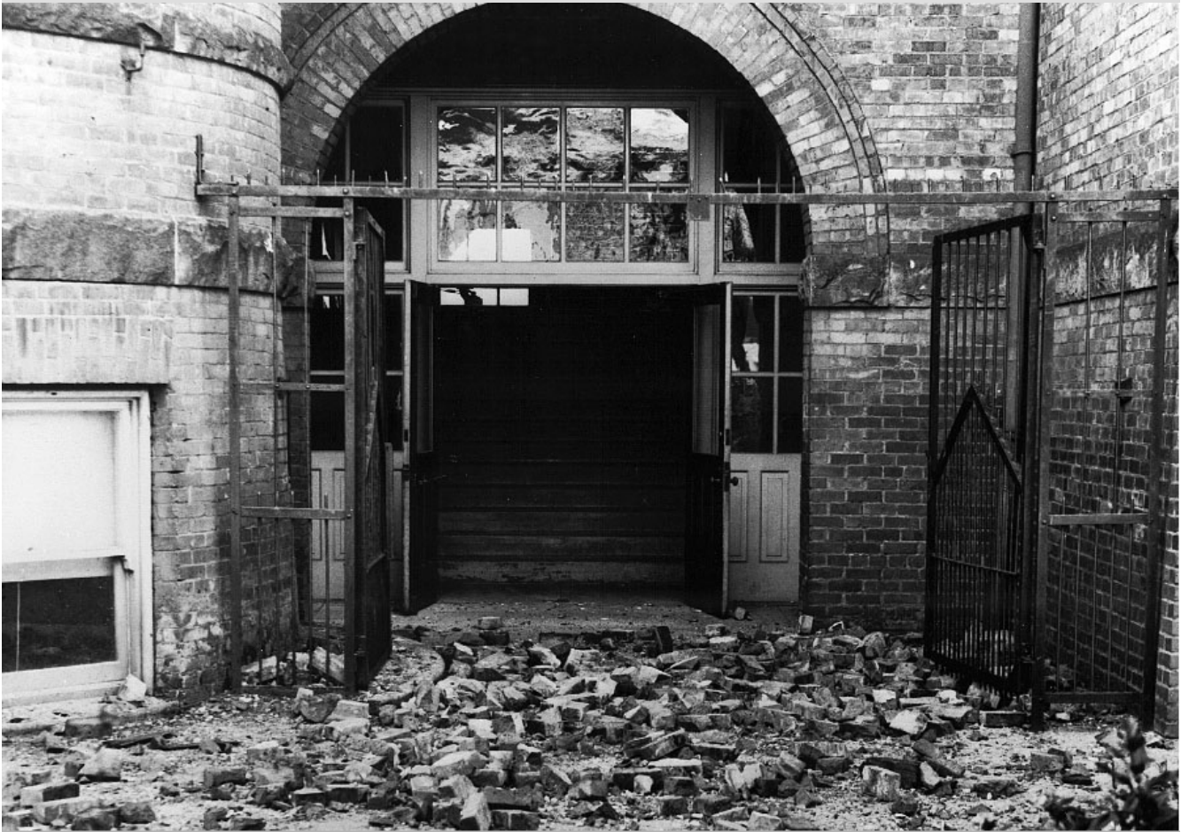
Figure 12-2. Close-up of an entrance to Lafayette School in West Seattle, covered with bricks that fell from this unreinforced masonry building during the 1949 Puget Sound Earthquake. Fortunately, the school was not occupied at the time, and no children were killed or injured. Damage to this and other schools in the 1949 and 1965 earthquakes led to a major retrofit of school buildings that minimized school damage in the 2001 earthquake. Photo courtesy of Washington Division of Geology and Earth Resources.
