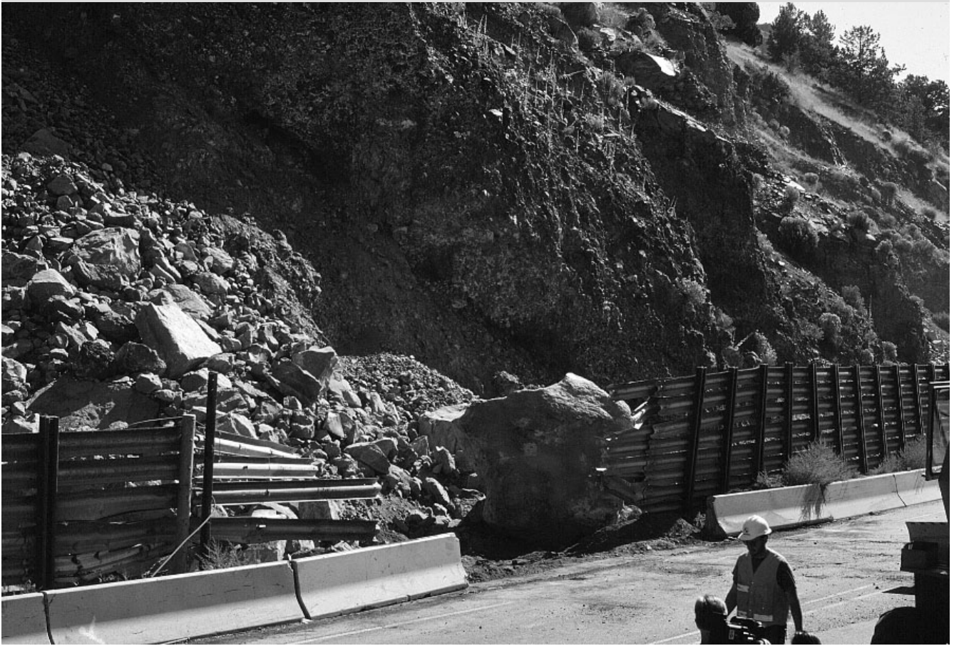
Figure 6-24. Boulder at Modoc Point, alongside U.S. Highway 97, that breached a roadside barrier and took the life of Ken Campbell during the September 20, 1993, Klamath Falls Earthquake. Boulder has been pushed back behind barrier.
