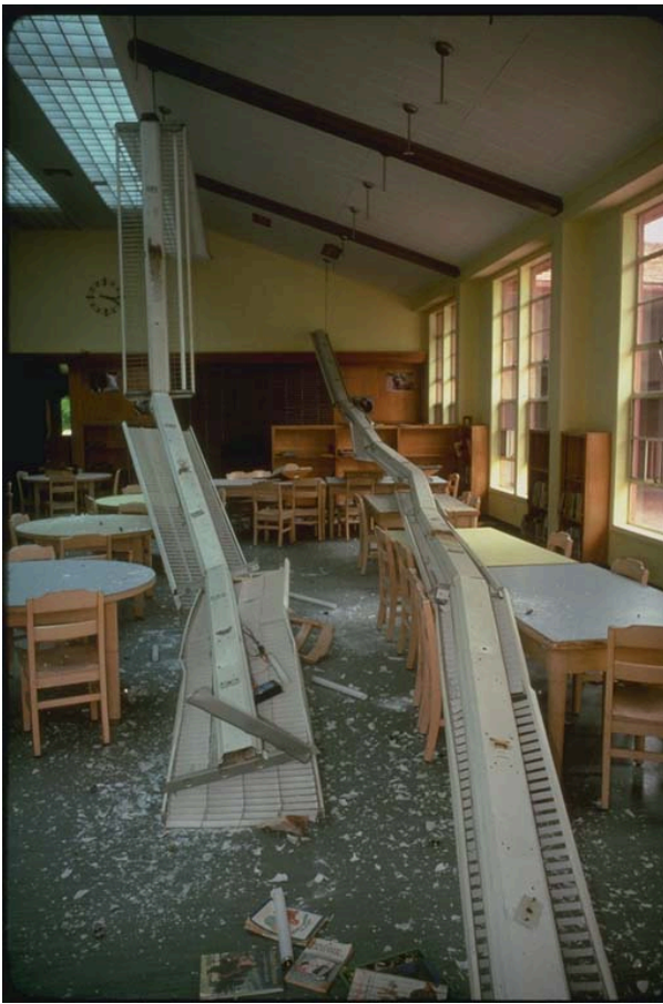
Figure 12-7. Failure of hanging light fixtures at library of Dawson Elementary School in California, fortunately unoccupied at time of earthquake. Note fallen ceiling tiles and plaster. Photo credit: Earthquake Engineering Research Institute
