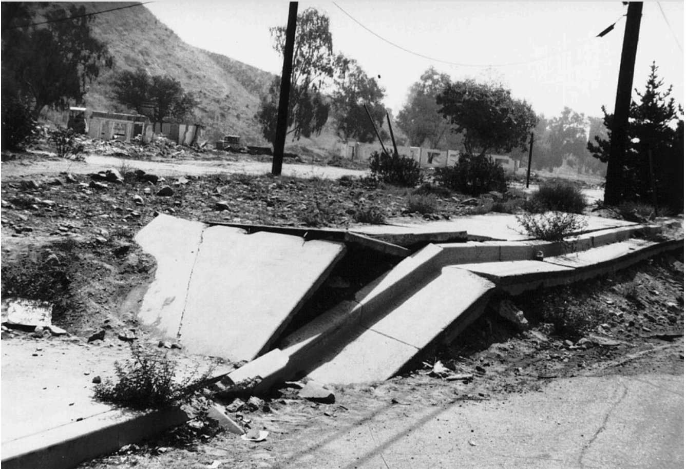
Figure 3-8a. Reverse fault in the San Fernando Valley, California, formed during the Sylmar Earthquake of February 9, 1971. Fault extends from left to right. Buckling of sidewalk indicates compression; fault dips away from viewer. Hanging wall (in background) was at same level as footwall (in foreground) before the earthquake. Ruined building in left background was part of a convalescent home in which several people died.
