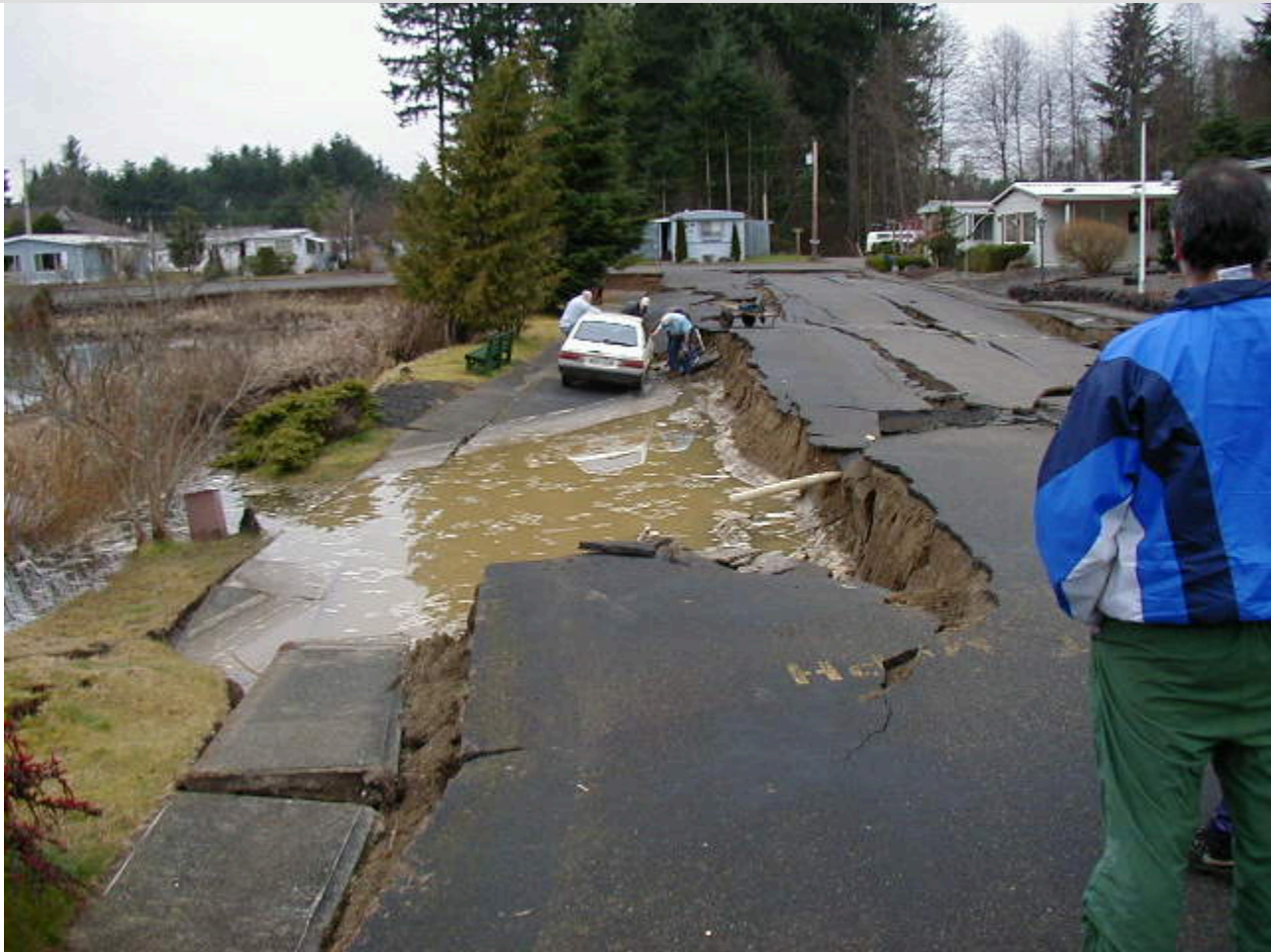
Figure 8-8. Lateral spread at Sunset Lake, Tumwater Memorial Mobile Home Park near Tumwater, Washington. Photo by Steven Kramer, University of Washington.
