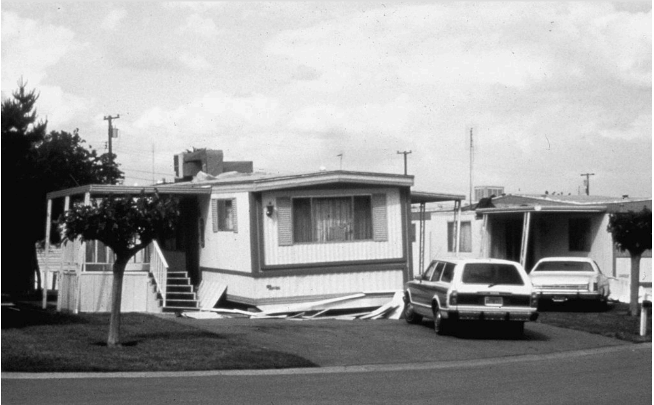
Figure 11-18. Mobile home has slid off its supports during an earthquake. Photo courtesy of California Office of Emergency Services
