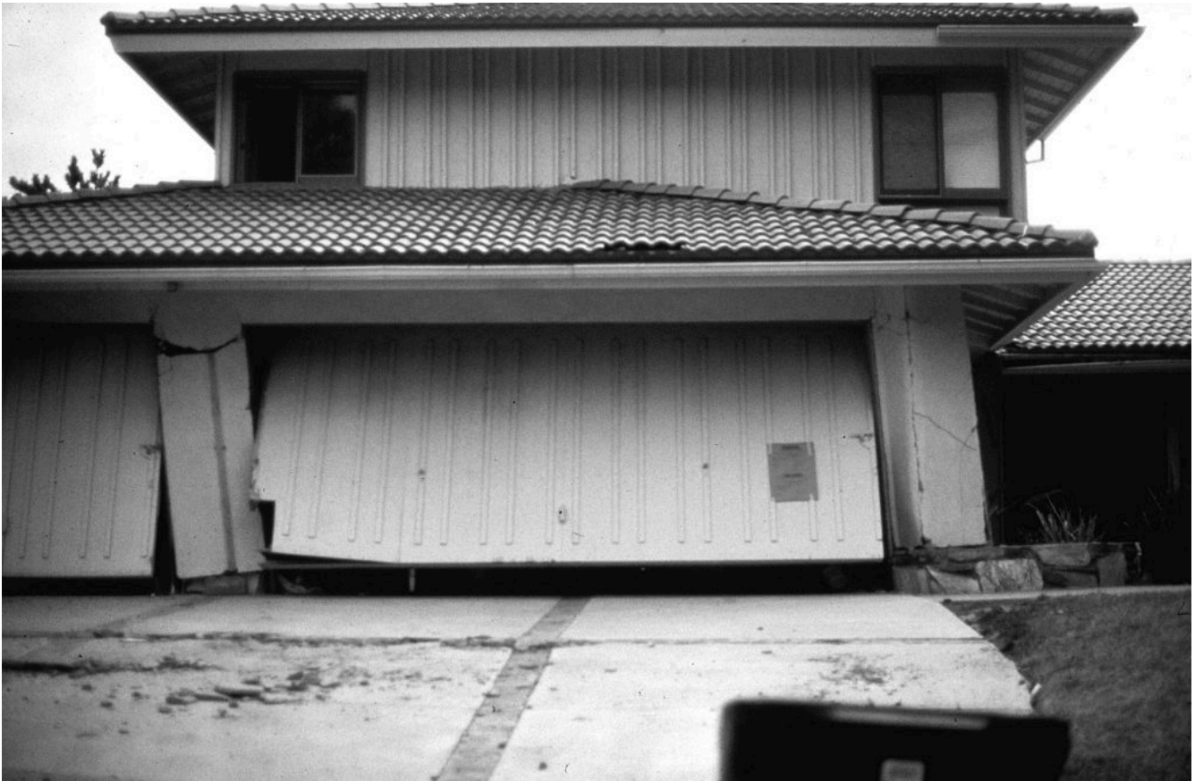
Figure 11-6. Soft-story failure to three-car garage during 1971 Sylmar, California, Earthquake. The large door opening resulted in inadequate shear resistance to horizontal ground motion. Photo by J. Dewey, USGS
