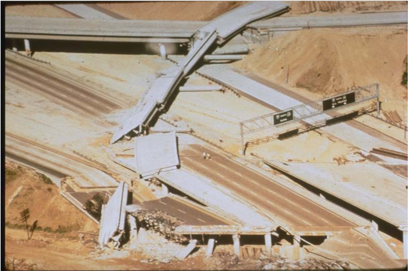
Figure 12-14. Damage to the Golden State Freeway (Interstate 5) and Foothills Freeway (Interstate 210) as a result of the 1971 Sylmar, California, Earthquake. Photo by E. V. Leyendecker, USGS
