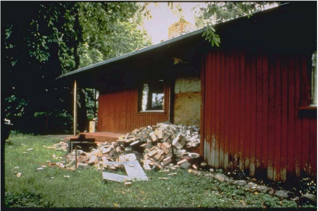
Figure 11-13. Brick chimney on this house in Petrolia, California, collapsed during the 1992 Cape Mendocino Earthquake. Photo courtesy of National Oceanic and Atmospheric Administration
