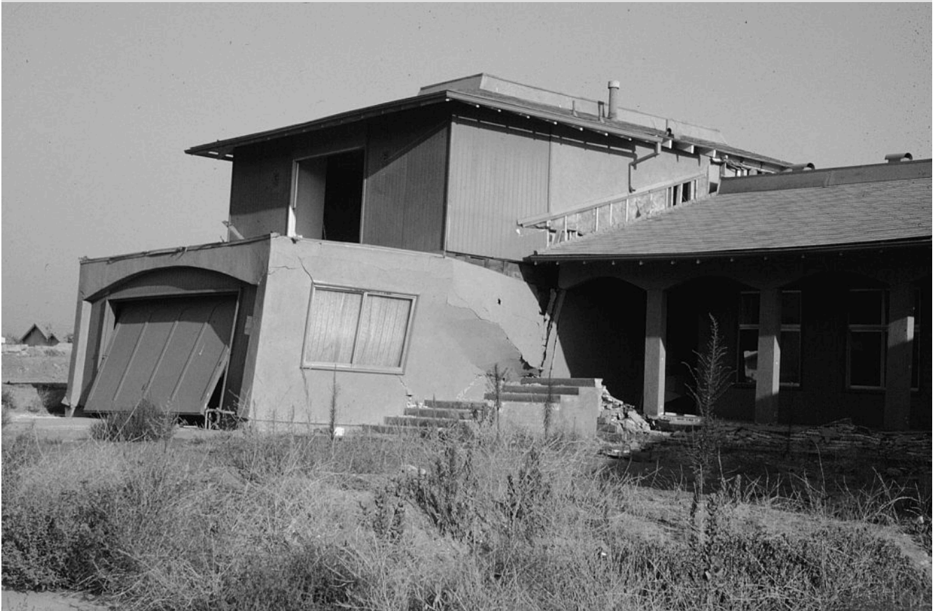
Figure 11-16. Split-level house in Crestview Tract, San Fernando Valley, showing failure of the connection between the single story (right) and the two-car garage with bedrooms above. Note the difference in height between the front steps and the single story, indicating cripple-wall failure of the single story. Photo by Robert Yeats
