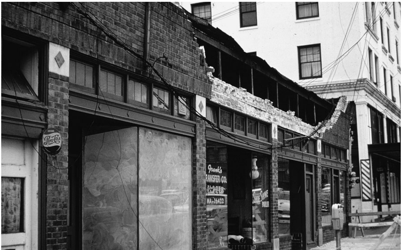
Figure 5-6. Falling bricks from this building on King Street, Seattle, during 1965 earthquake caused one death. From Karl V. Steinbrugge Collection, Photo 2876
