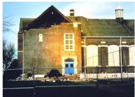
Figure 14-3. Damage to Molalla High School, an unreinforced-masonry (URM) building, from the Scotts Mills Earthquake of 1993. Bricks from the URM gable over the doorway fell on the steps and sidewalk. Fortunately, the earthquake occurred early in the morning, and no students were in the building. Photo courtesy of Yumei Wang, Oregon Department of Geology and Mineral Industries
