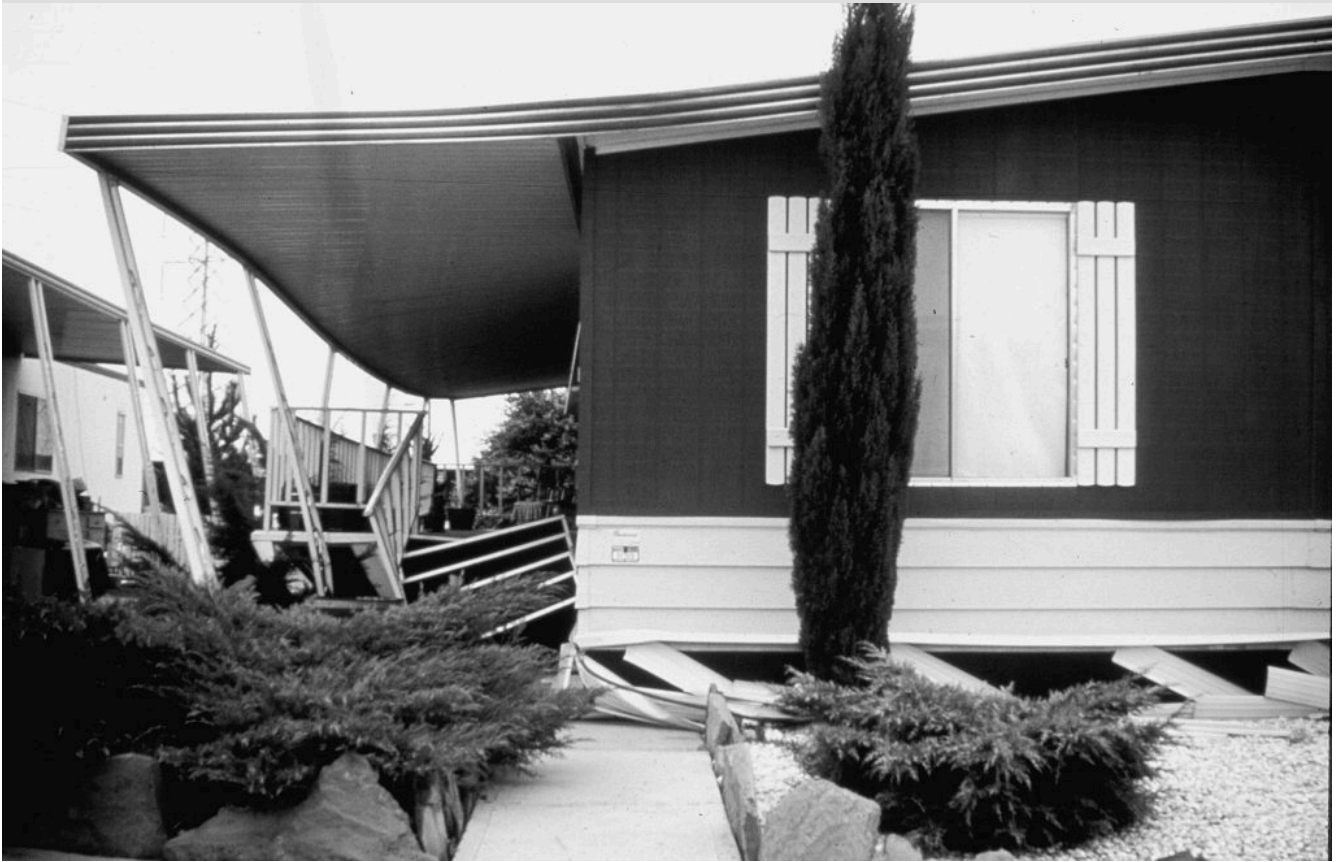
Figure 11-17. This manufactured home slipped off its supporting piers during an earthquake. This type of failure can be avoided by bolting the house to its foundation, as is required for other houses in most states. From Karl Steinbrugge Collection, University of California at Berkeley
