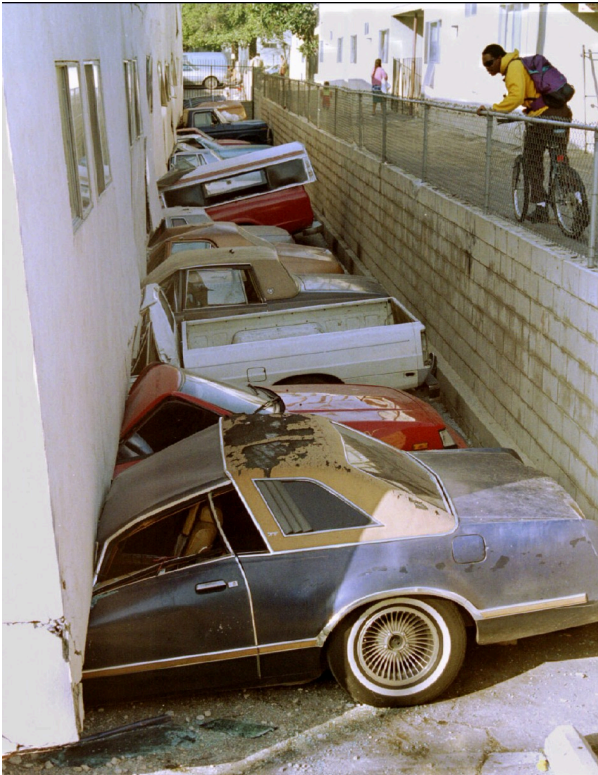
Figure 12-12. Soft-story problem in apartment building where bottom floor is the garage. During 1994 Northridge earthquake, the garage acted as a soft story, and the apartments above collapsed down on the cars.
