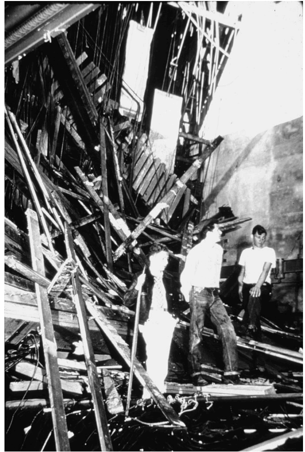
Figure 5-3. Puyallup High School damaged in 1949 earthquake. Unanchored roof and ceiling beams over the stage of the auditorium slid off supporting walls and crashed to the floor. From Thorsen (1986); illustration from collection of Washington Division of Geology and Earth Resources
